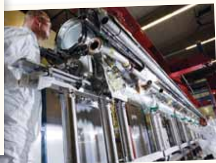
Before the resonator string is installed in the accelerator module, other important elements, such as helium lines, are added.
