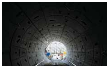
The future experimental hall and one of the tunnels for the European XFEL
