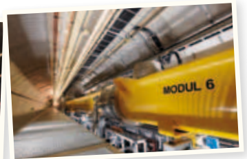
The finished modules are installed in the accelerator tunnel.
