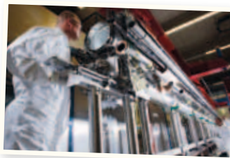
Helium lines and other components are fitted into the module.
