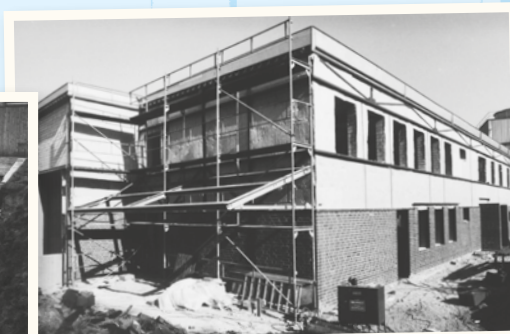
Construction of the HASYLAB experimental hall
