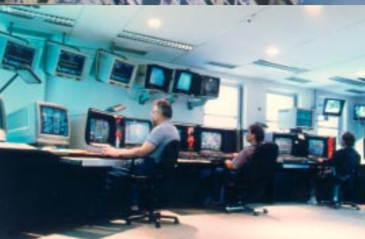
In the control room of the HERA refrigeration plant
