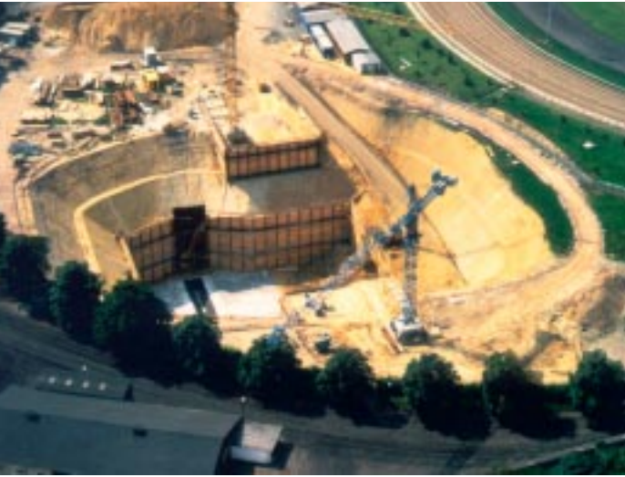
The four underground HERA halls were constructed by open excavation.
