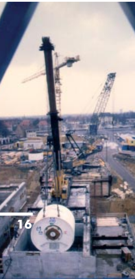
The tunnel boring machine HERAKLES is lowered into HERA's South Hall.
